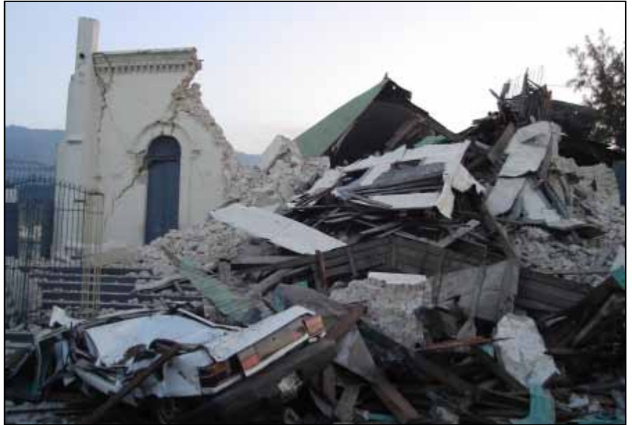
Church of Santa Ana, in which the brothers of the Fraternity of St. Alexander serve. The presbytery was also damaged and here the pastor was killed.
