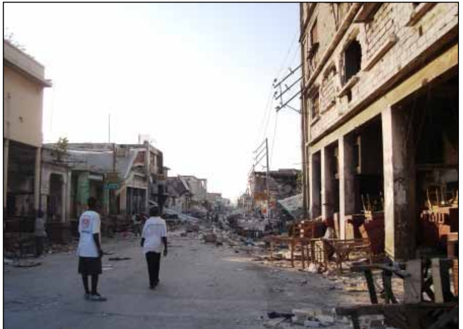
The commercial area of Port au Prince
