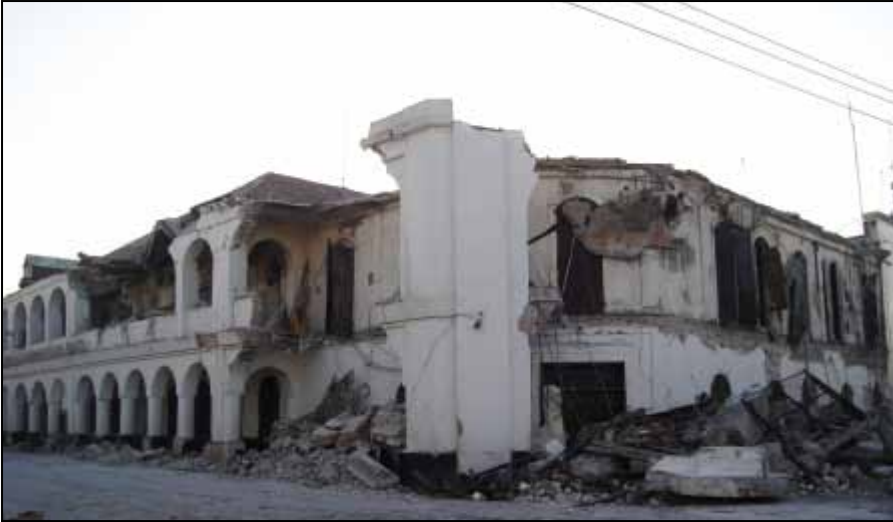
Building of the Electricity Authority.
