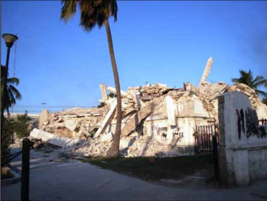
Mayor's office of Port au Prince
